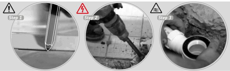
Secure in place and connect the waste outlet. Always clear away all excess adhesive. Support the bottom of the waste. **Step 5.** The edges of the SureForm must finish flush and level with the top of the finished screed top surface which should also be level. Ensure the fall is correct and the former is level before allowing to dry.
