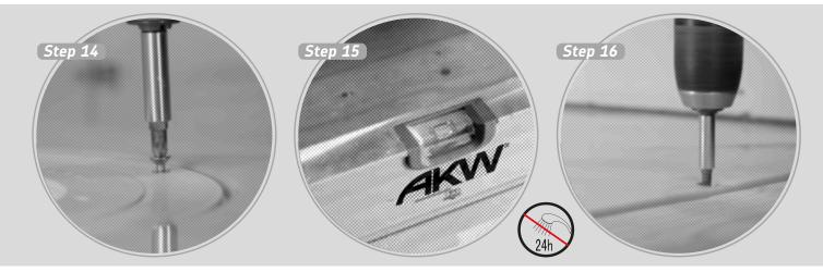
**Step 16.** Fix down – only when the former is fully supported and level with the surrounding floor, apply an adhesive or mastic to all supporting surfaces and screw down the edges of the former onto the joists and noggins. Foam should not be used as a load bearing support as it will break down under repeated product use. Do not overtighten the screws.
